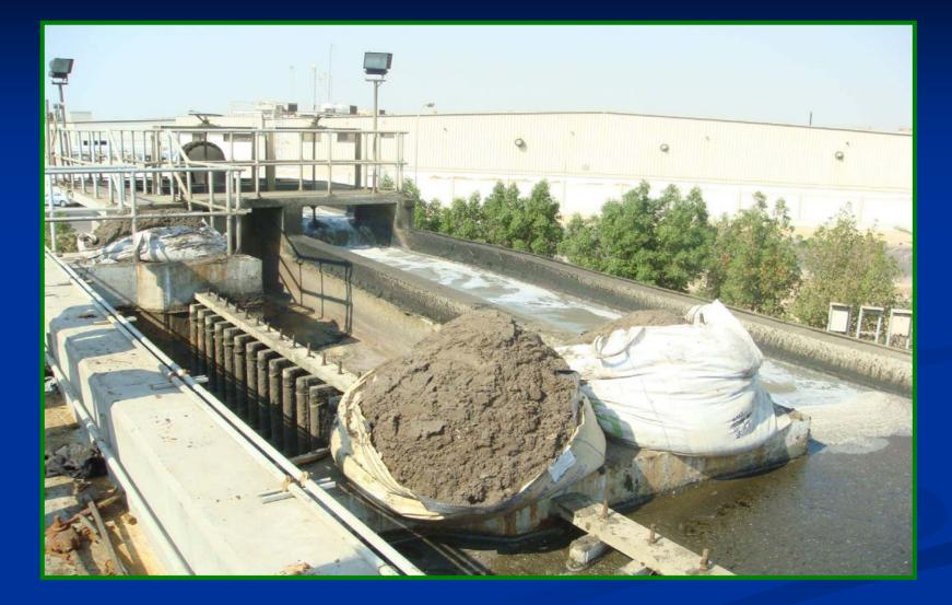
**Excessive Sludge Accumulation in Inlet Works**
