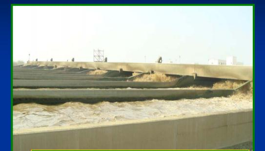
No. of Aeration Tanks = 2 Total Volume = 65,000 m<sup>3</sup> Total No. of Aerators = 10 Total Power = 1200 KW
